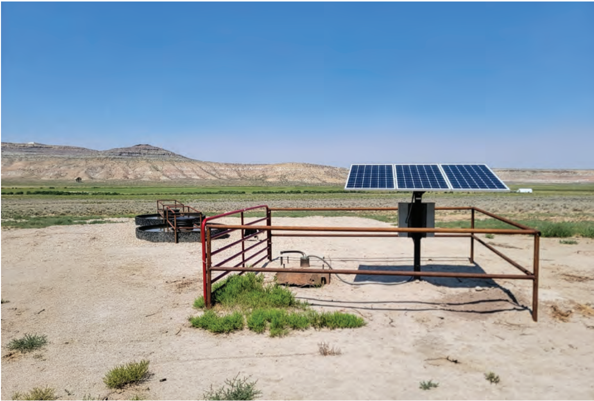
Sublette County Conservation District installed a solar-powered well pump and tire tanks to provide water for cattle. The location of these tanks improves range conditions by better distributing cattle across a grazing allotment.
