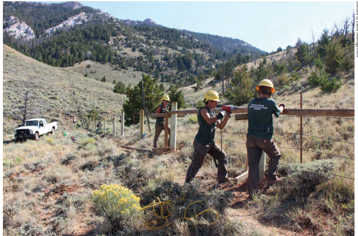
A Montana Conservation Corps crew converts old barbed- and mesh-wire fence to wood post, rail-top, and wire fence on Ferris Mountain.
