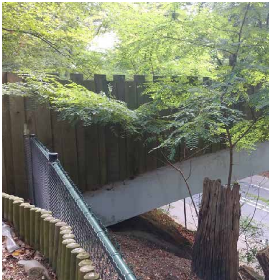
A bridge made from fiber reinforced polymer allows small wild animals to cross safely over a highway near Grebbeberg, Netherlands.
